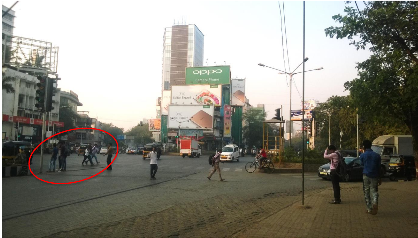
Lack of pedestrian refuge
