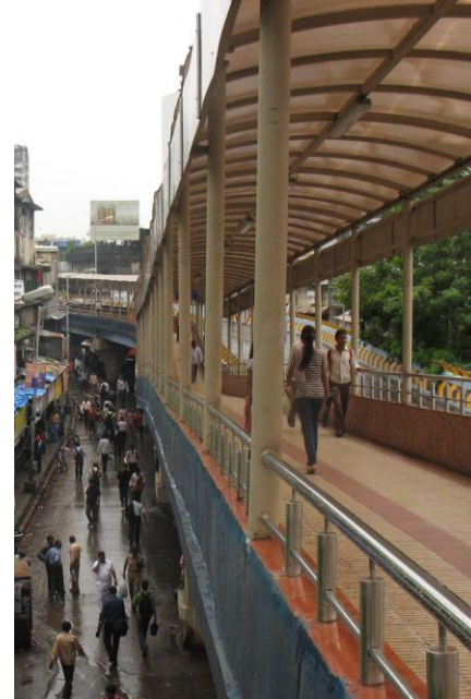
Grade separated skywalk at Thane station India (WRI India)
