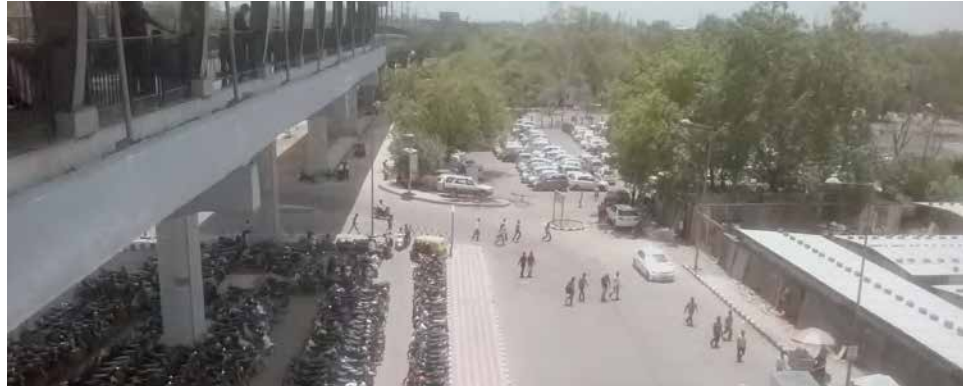
Park and Ride facility at Chattarpur Metro Station Parking, Delhi, India
