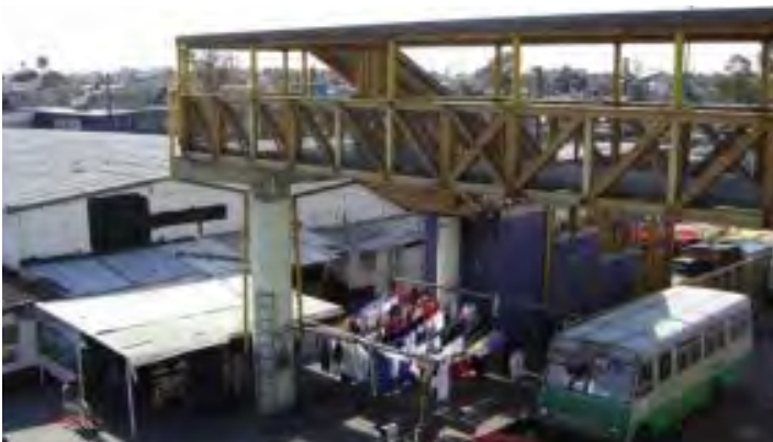
Tepalcates Central Station (Before)
