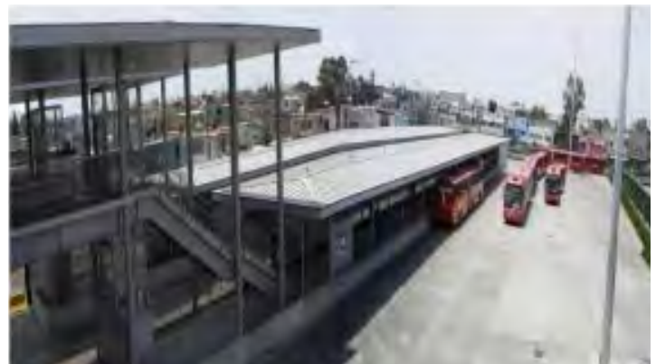
Tepalcates Central Station (After)
