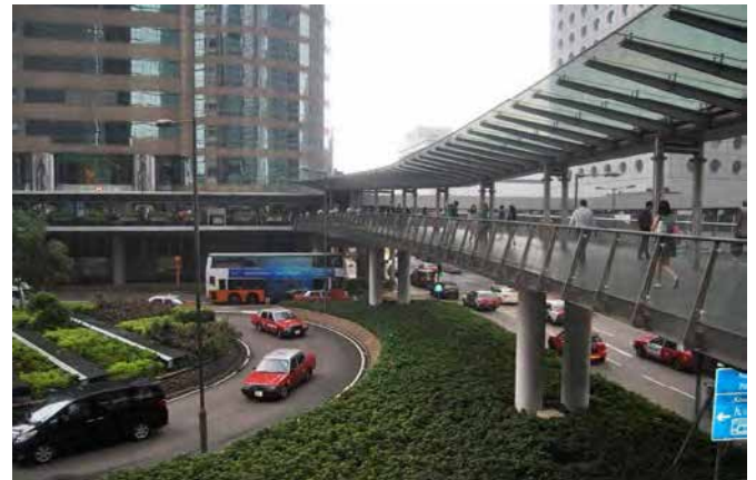
Sky-walks in China SAR connecting commercial and business destinations to transit stations (Source: © WRI India)
