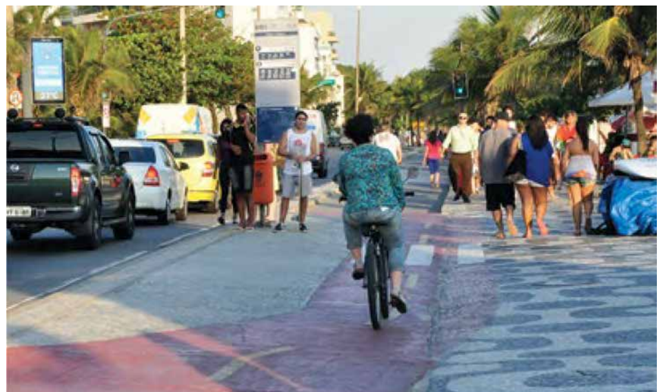
A bus station bypass in Rio de Janeiro, Brazil that raises the bicycle lane to the sidewalk level while bypassing the bus waiting area. (Source: © WRI)
