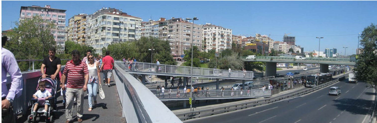
Elevated pedestrian bridges to Metrobus
