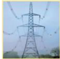
Karnataka Electricity Governance Network
